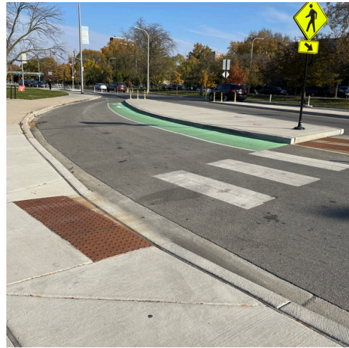
ID: Photo of the drop-off area with cut curbs for access.
