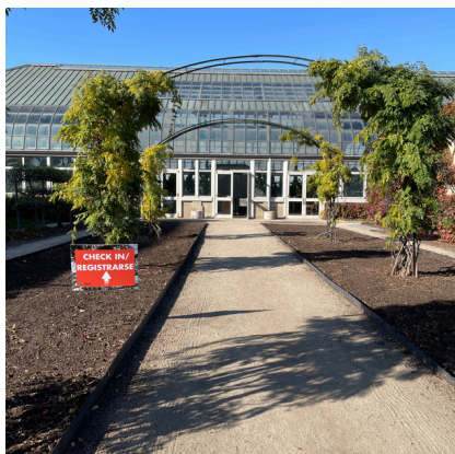
ID: Photo showing the temporary entrance from the outside.
